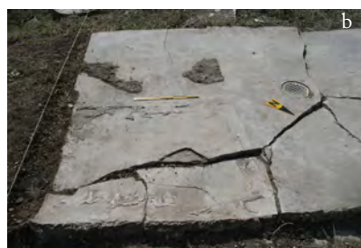
Fig. 19. C20: space with floor drain and washing installation.
