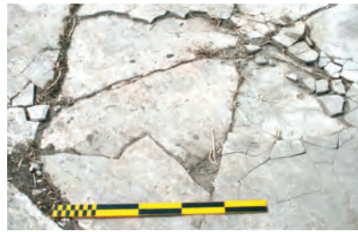
Fig. 42. C20: screed degradation.
