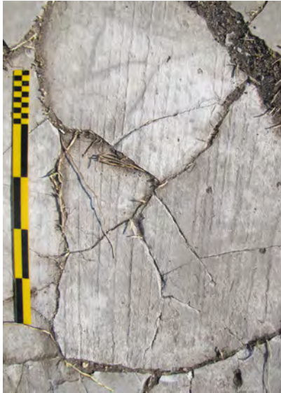
Fig. 41. C20: screed levelling marks.
